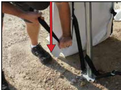
19. Locate the fourteen X-Bracing straps (HT531), 148" (370 cm) in length. On each corner and side tee fitting take the loop end through the 1¼" (3.175 cm) welded D rings on either side of the hip/rafter poles, run the rest of the strap through the loop, and pull tight.
