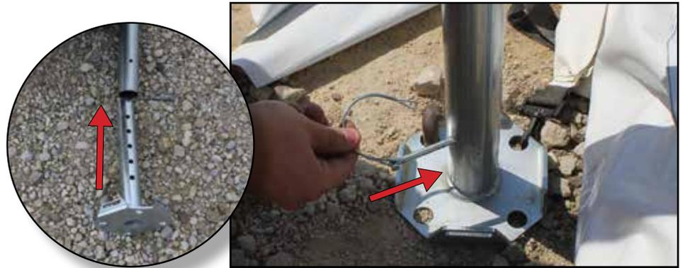
9. Lift one side of the frame up and slide the legs (Green/HT2GST80) with base plates into the bottom of the two corner fittings (F01CORHT) and pin using pin and bail (HT570). Slide the pin through the hole in the corner fitting and leg hole then connect the bail end around the pin.
