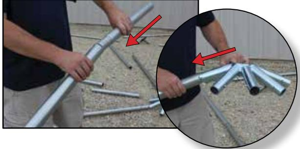
3. Take the combined hip rafter poles (Green/HT2GST80) and slide onto the remaining post slots on the 8 way crown (F048WCHT). Lining up the holes until the push pins engage.
