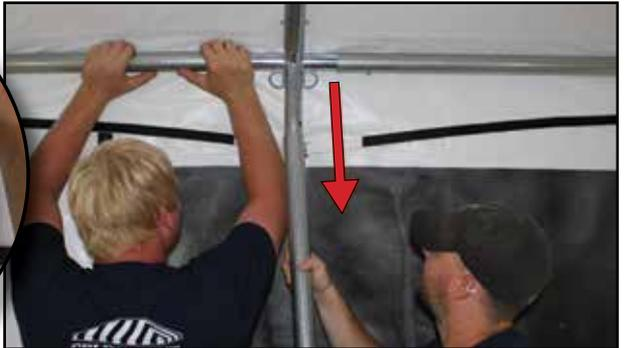
7. On one side remove both legs with base plates from the corners, place off to the side, and carefully set the frame down.
