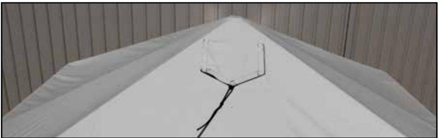
31. To use the floor as a liner first flip the floor upside down so the D ring, which is in the middle of the floor, is facing up. Tie a rope or a string (not included) to the D ring. Hang the D ring two-three feet below the center of the 8 way crown. Attach the spring snaps to the D rings on the fitting or to the wire bail on the pin and bails.
