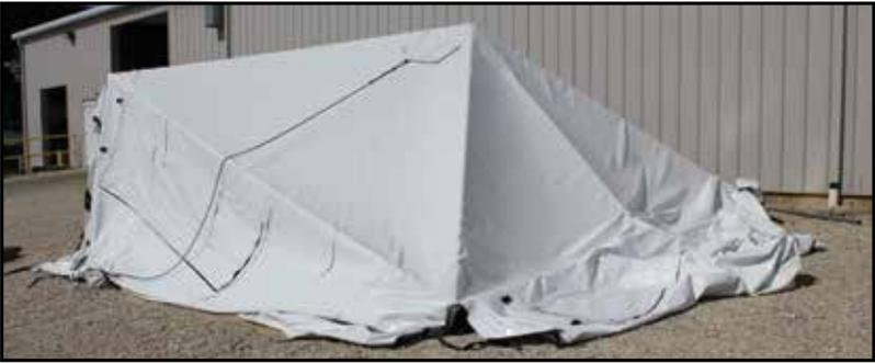
8. Remove the other two corner legs and base plates, place off to the side, and carefully set the frame all the way down.
